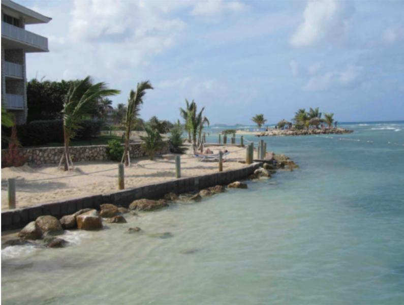
Figure 2. Structural protection to preserve artificial beach area.
